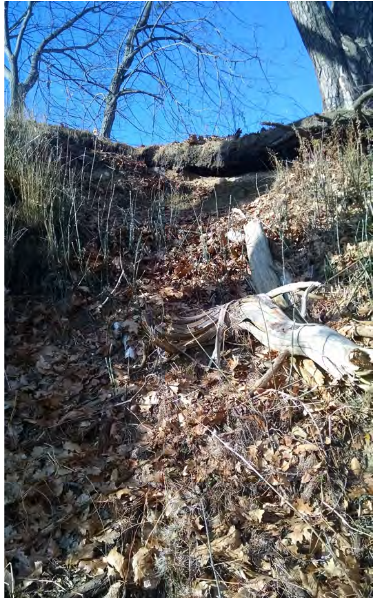
Figure 3. Removal of upland vegetation increases erosion at the Mackworth Island sites.
