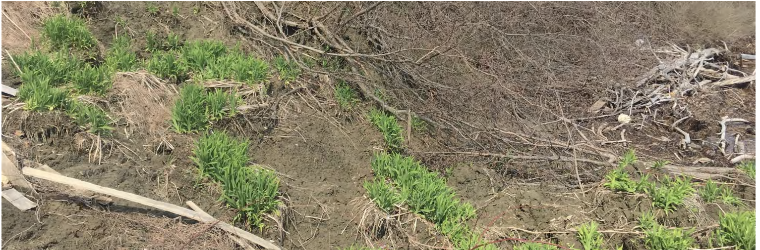
Figure 4. Plant additional woody and herbaceous planting throughout the terraces of the failure.
