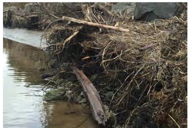
Figure 1. Root wads inserted into unstable banks can help protect bare soil from erosion, from a project in coastal Oregon. In areas not suitable for living shorelines, root wads can be an effective alternative providing stabilization and habitat.
