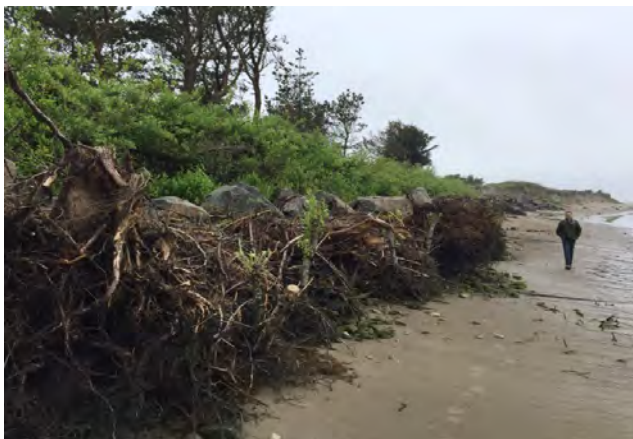
Figure 1. Root wads inserted into unstable banks can help protect bare soil from erosion, from a project in coastal Oregon. In areas not suitable for living shorelines, root wads can be an effective alternative providing stabilization and habitat.
